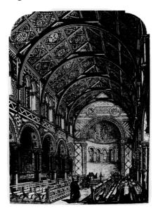
As the Chapel is situated above the Great Hall, Scott had to overcome a number of structural difficulties. He had to use a light-weight construction system for the arcade and upper nave walls that concentrate the loading above the iron columns on the floor below. The wall is therefore fabricated in iron with paired ornamental cast iron columns and an applied timber frame facing above. The original pitched roof was lightly built, in order to reduce stress on the wall framing.
