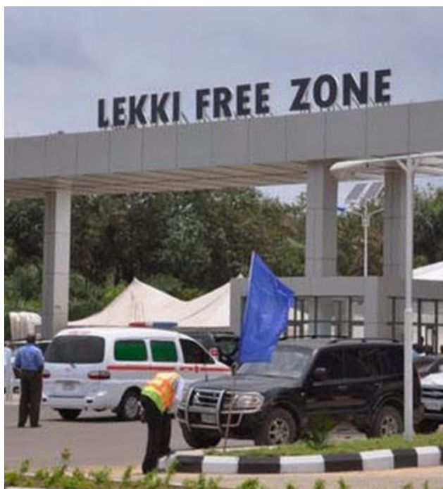
Image 8.1 Lekki Free Zone gateway. Source: Author’s photograph
